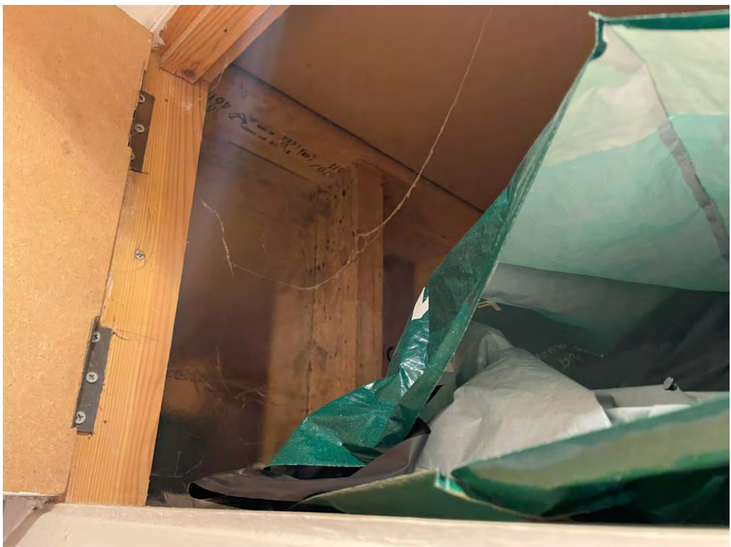
Figure 33: Modern wall to be removed, room 22.
