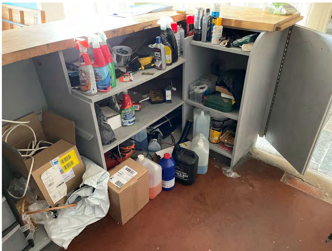
Figure 31: View behind the existing bar. Plywood construction is clear.
