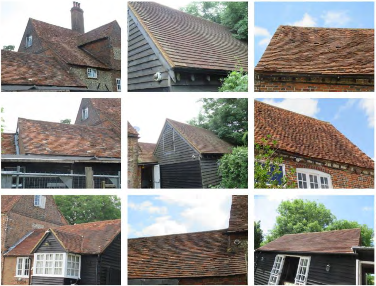
Pitched roof sections
