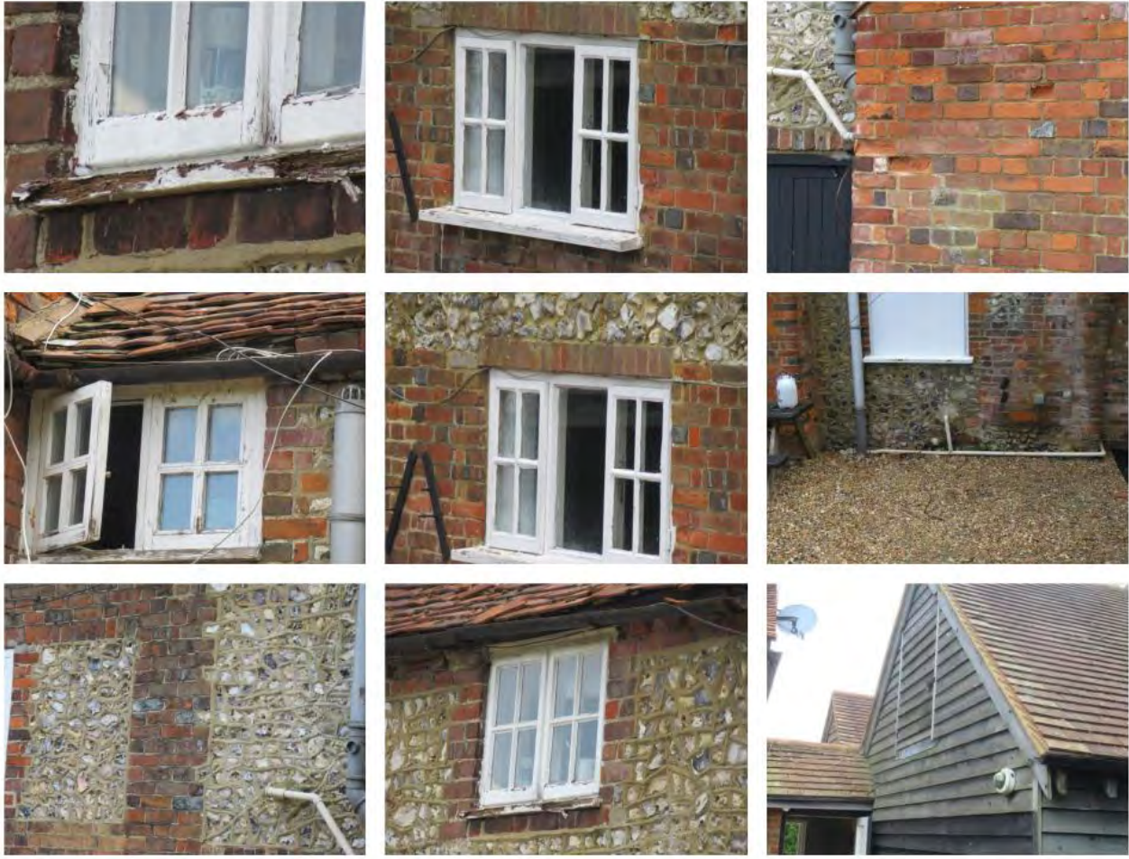
Rear elevations – detail
