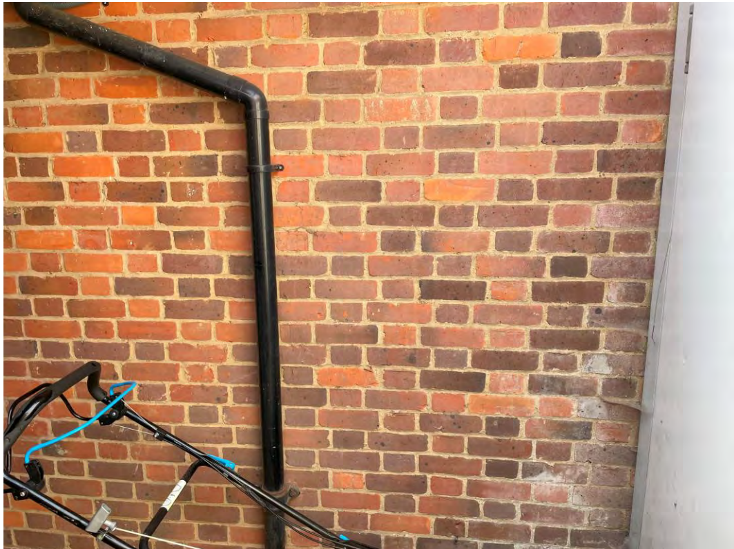
Figure 13: Rear of front section of north extension. Brickwork is modern.
