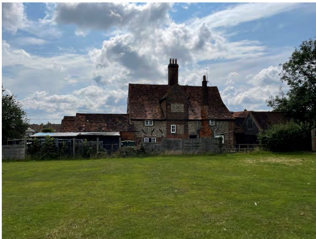
Figure 24: Rear elevation of the King William IV Public House. As seen from the playing fields.
