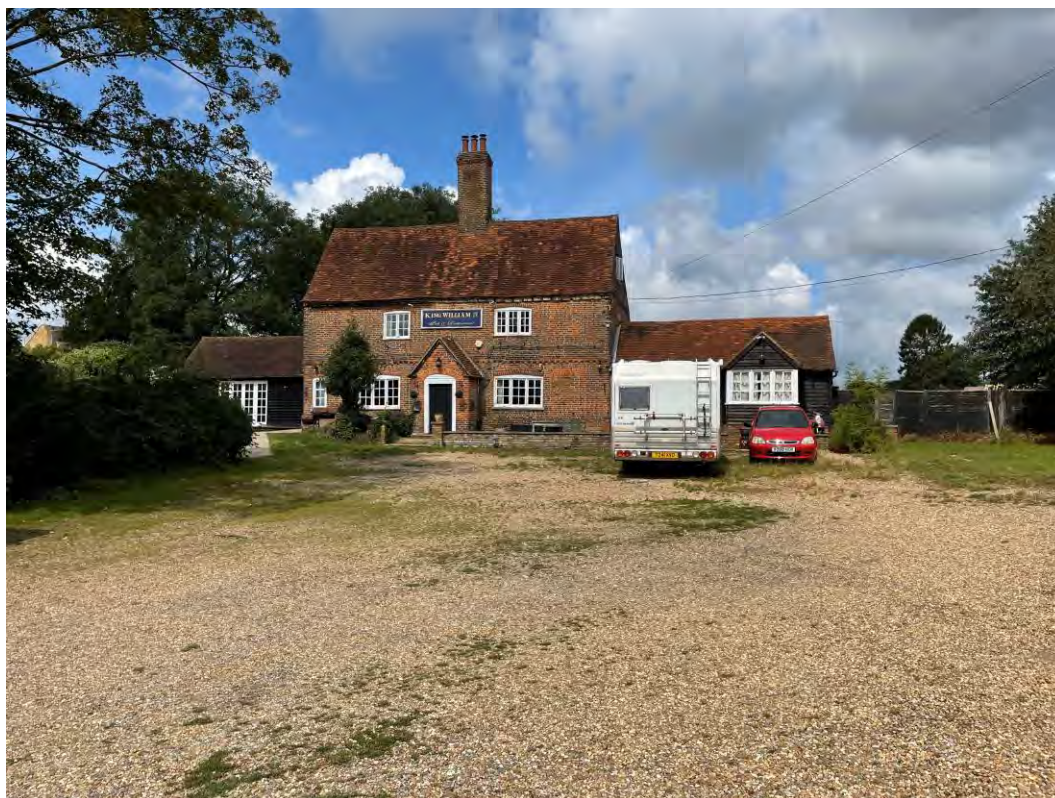
Figure 26: Car park in front of the listed building.
