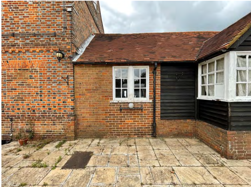
Figure 12: Front elevation of north extension. Brickwork has been rebuilt.
