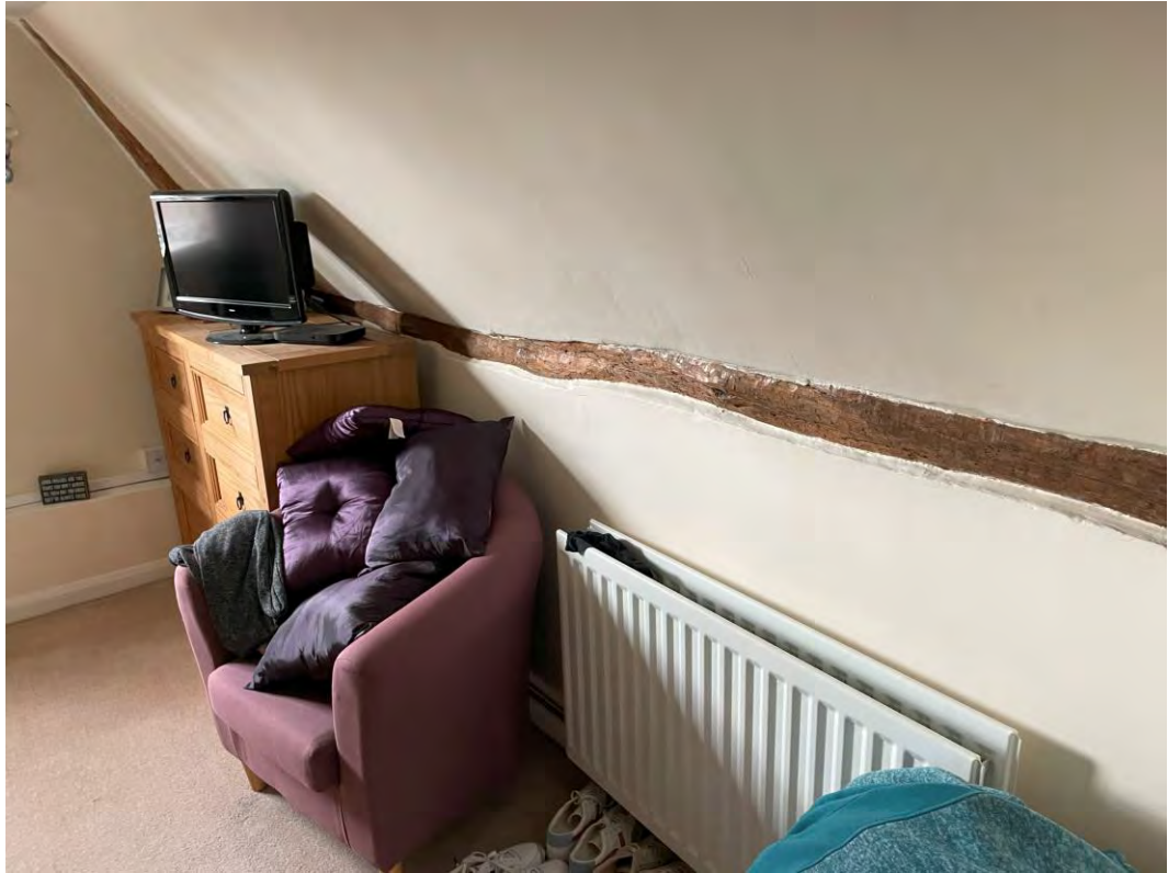
Figure 23: Timber roof structure, visible on second floor.
